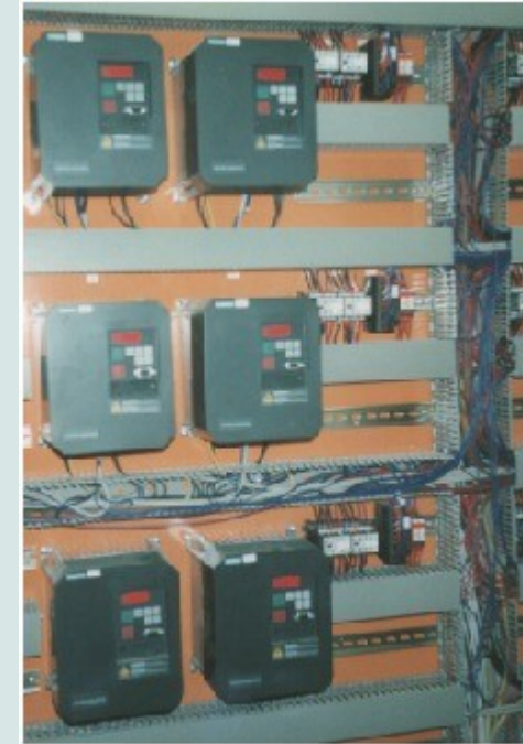
Poor EMC Installation: all wiring mixed.
