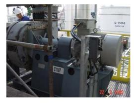
2. Changing the old VSD 30 kW to new "SIEMENS" MM430 VSD 55 kW and Installation with new control Panel.
