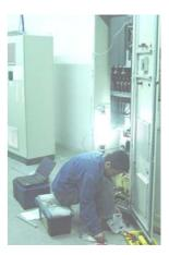
3. Design / Installation / Commissioning "SIEMENS" VSD 55 kW and Installation with new control Panel.
